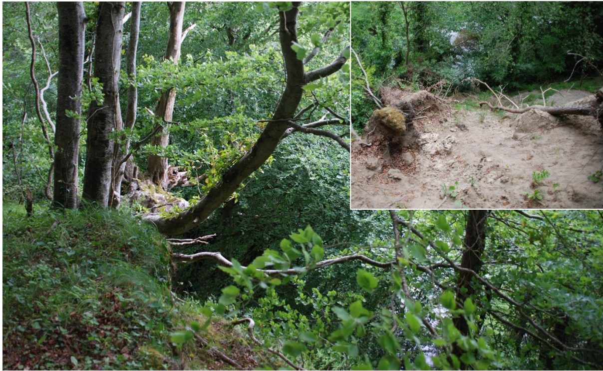
Plate 1: Proposed works area (main image) and slippage area (inset).
